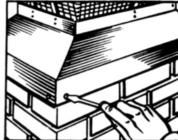
DO NOT OVER TIGHTEN STUDS It is only necessary to tighten the points in securely against the masonry surface, leaving balance of screw protruding. Extend points of studs into mortar line or other indentation in the chimney, if possible.
